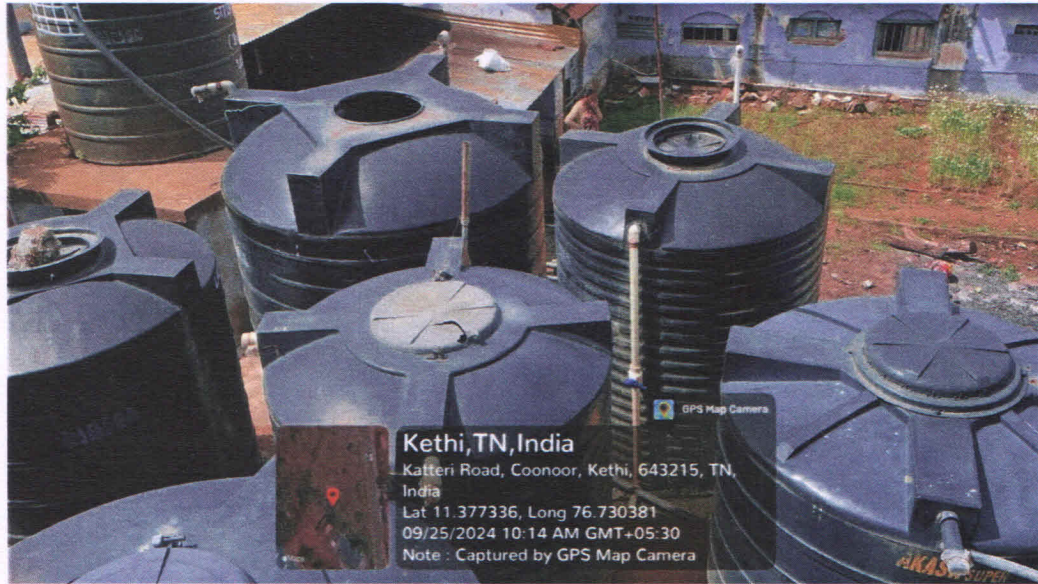
Top Of The Central Mess
